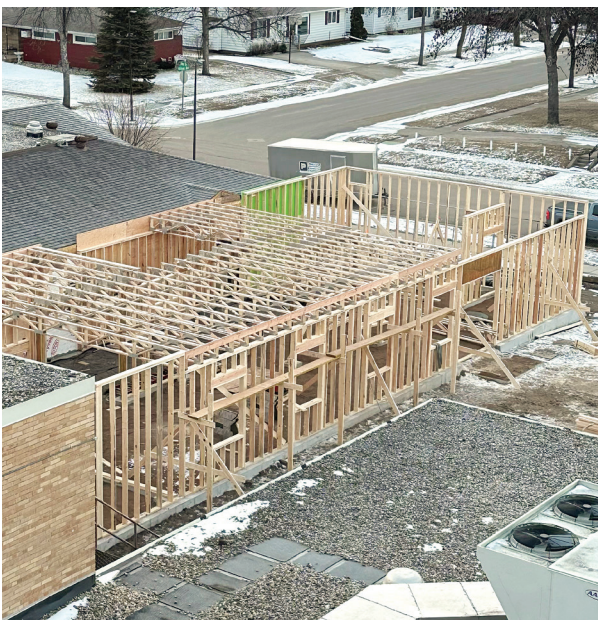
This picture taken Feb. 15 shows the actual clinic expansion construction.
