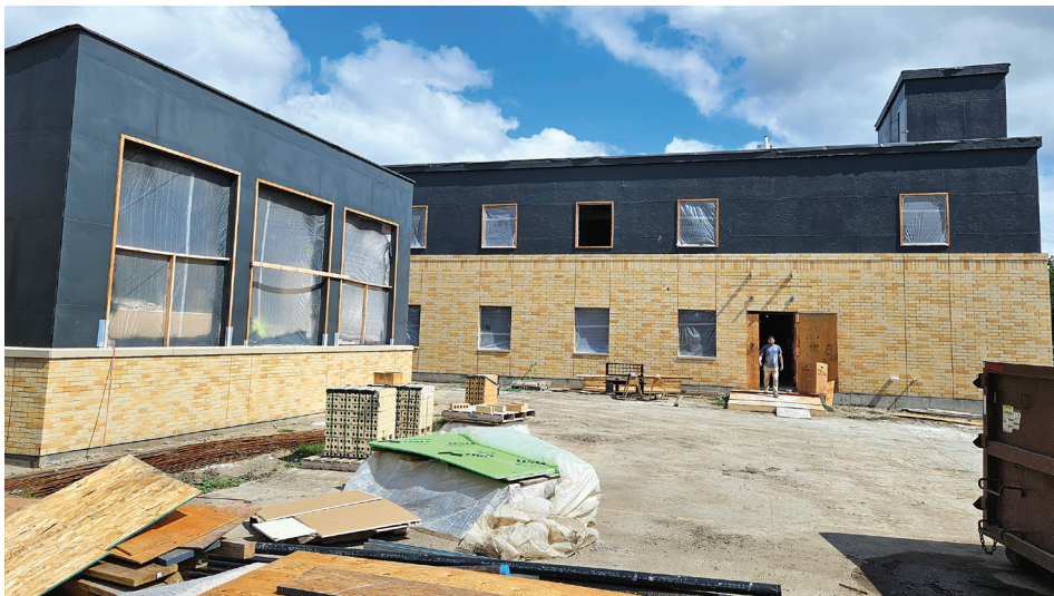
Exterior of dining (left) and clinic (right) expansion.
